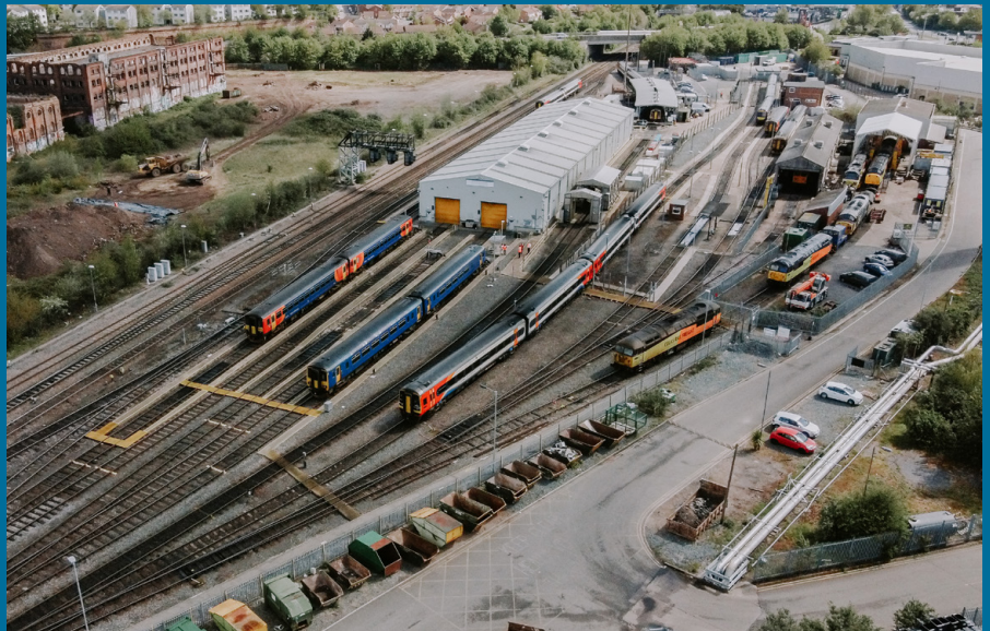
East Midlands Rail’s Nottingham Eastcroft depot.
